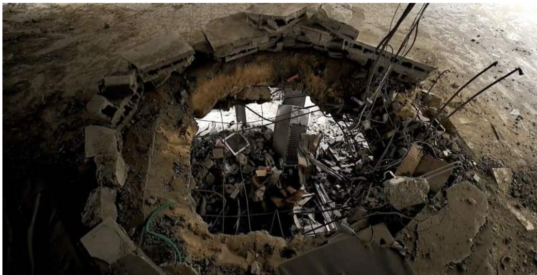
Figure 7. The hole from the 1st floor to the ground level of the building. Video source: Monitor/WDR.
