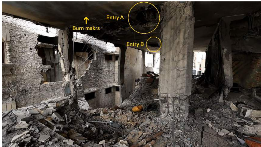
Figure 4. Annotated still image from video documenting the apartment shows the location of the two entry holes. Video source: Monitor/WDR.
