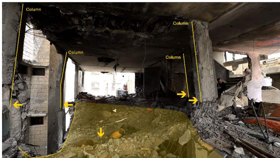
Figure 5. Annotated still image from video documenting the apartment shows burn marks on the ceiling as well as the way the columns and the floor are pushed outward. Video source: Monitor/WDR.
